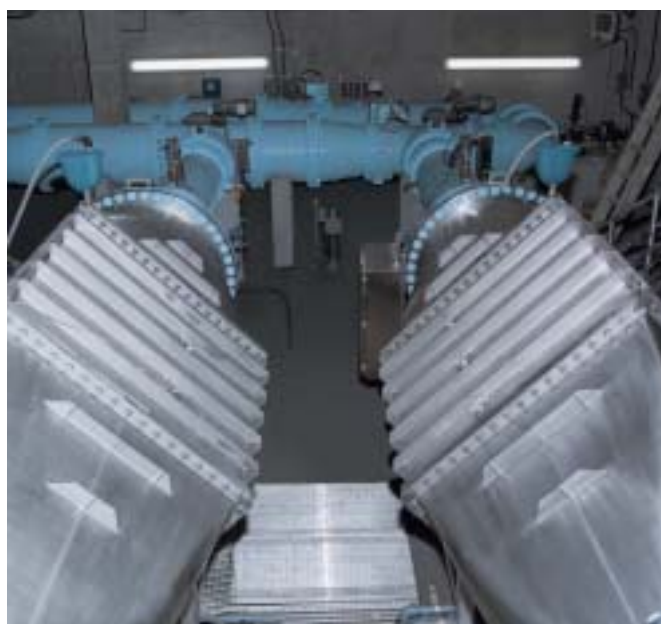
WEDECO UV System Type K for disinfection of drinking water in Clayton County / USA
