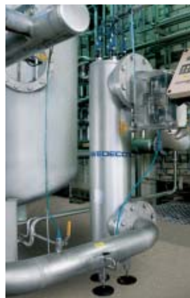
WEDECO UV installation for drinking water in Marheez / Netherlands
