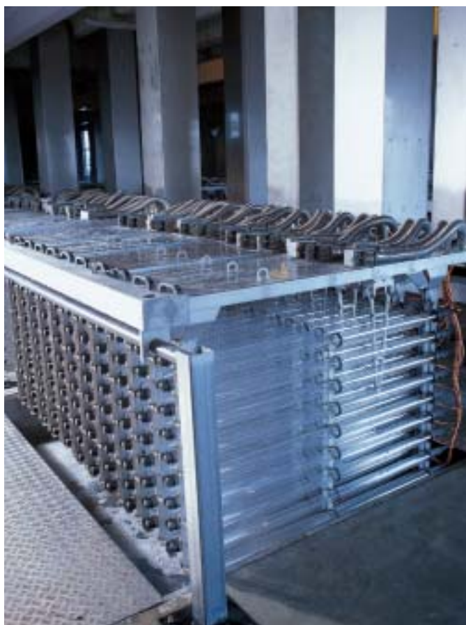
UV modules ready for maintenance in Manukau / New Zealand
