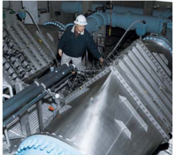
WEDECO K reactor as UV disinfection step at waterworks Weber Basin, Utah, USA
