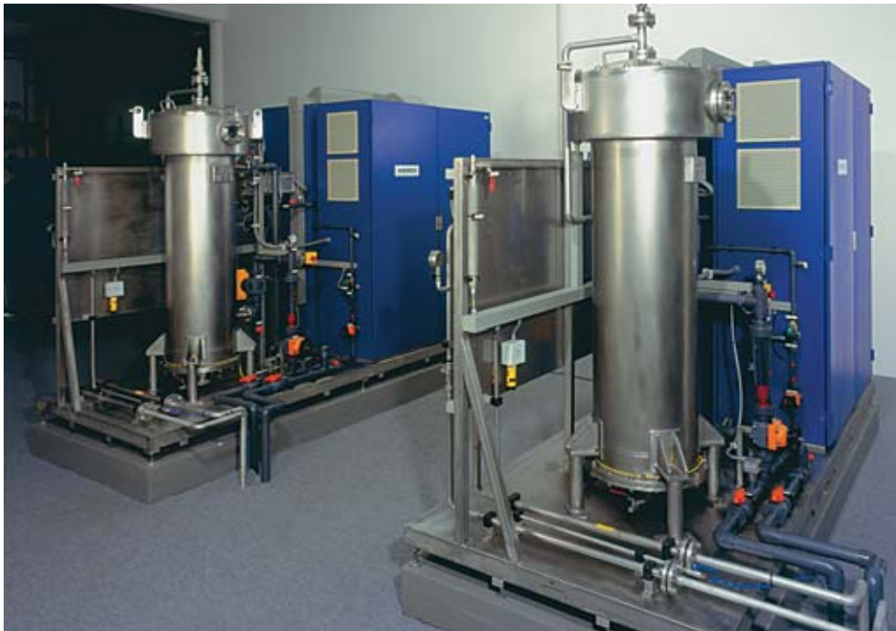
Ozone system for drinking water treatment „Am Staad“, Düsseldorf, Germany
