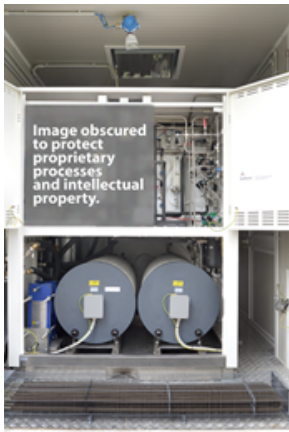
Two Electrolyser stacks in the Electrolyser unit.
