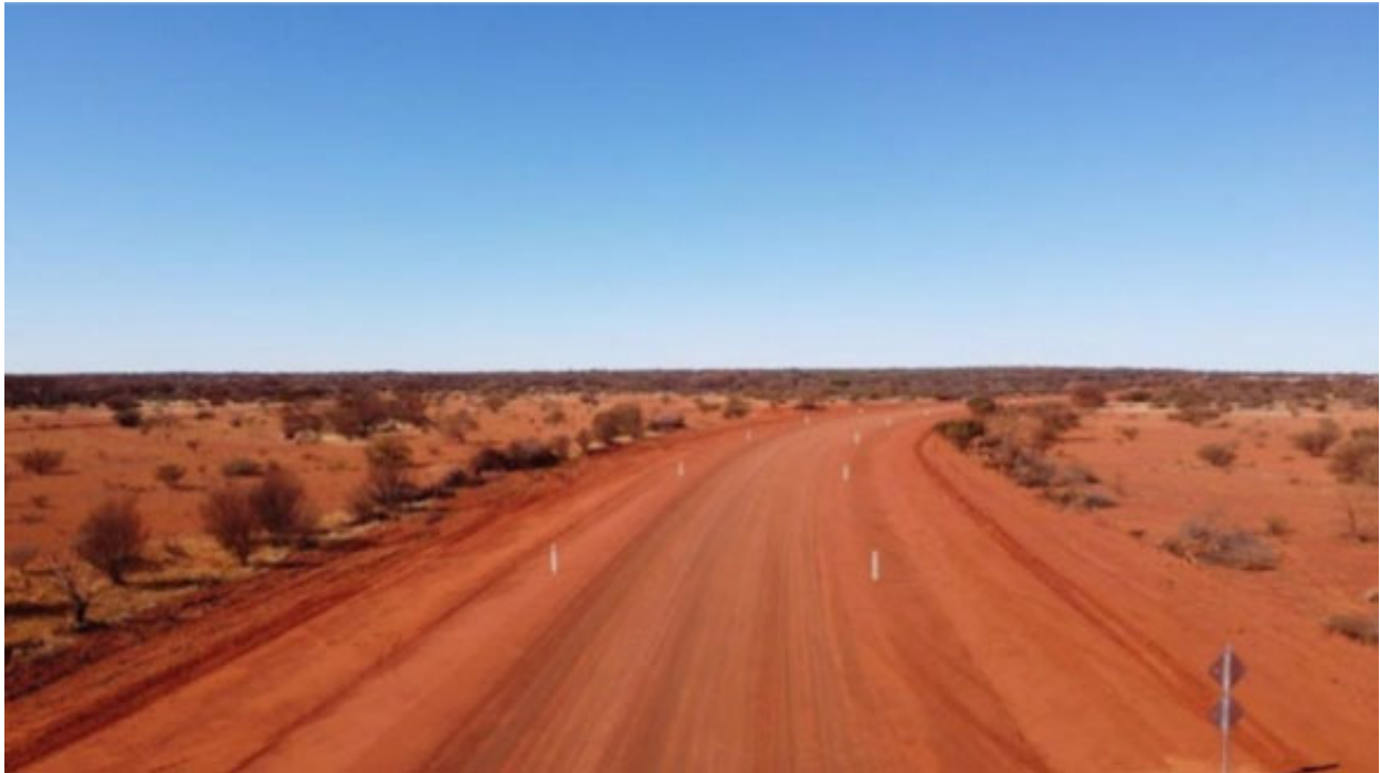
Plate 5-1 View of Approach Road to Karlawinda showing Physiography and Vegetation (Source: Capricorn 2020)
