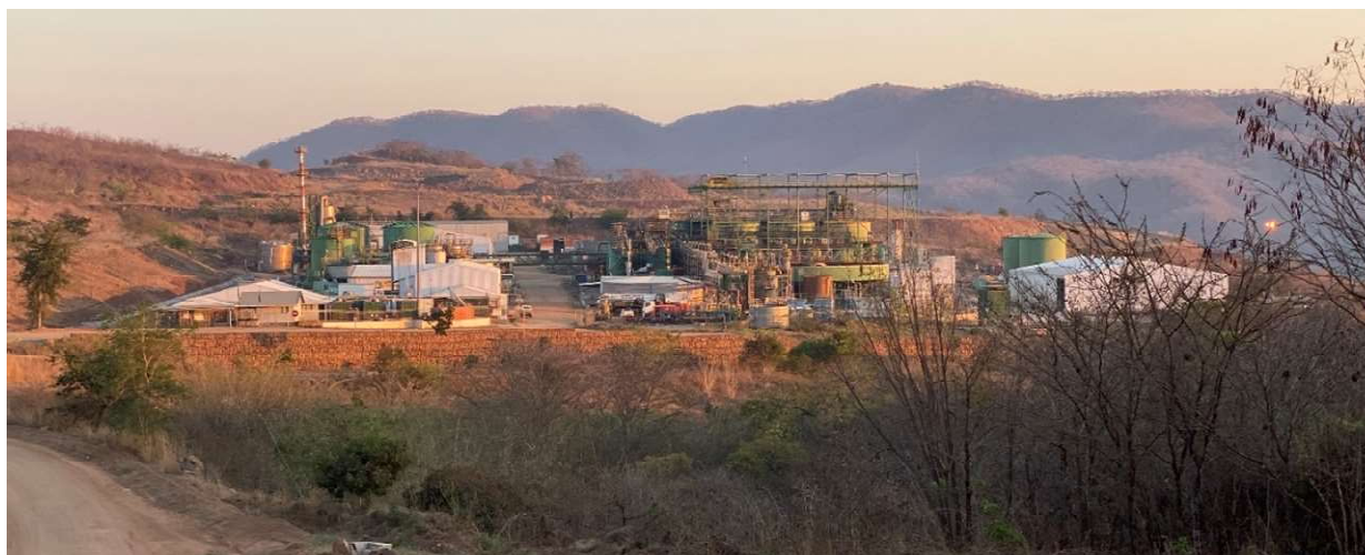
Figure 2: Kayelekera Process Plant and Surrounds – October 2019
