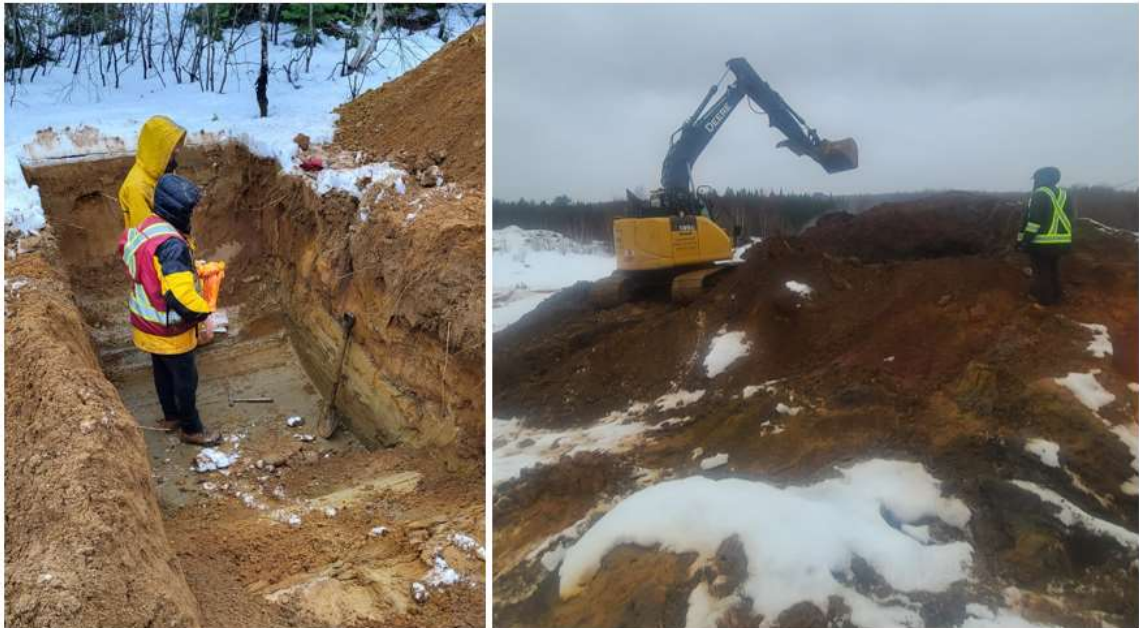
Figure 9.3: Typical test pit excavations
