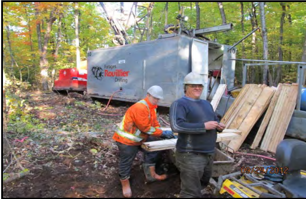
Photo 1: Drilling work in progress during 2012 exploration.
