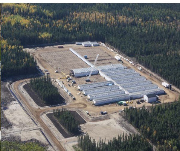
720 Bed Camp under construction near Fort McMurray, Alberta
