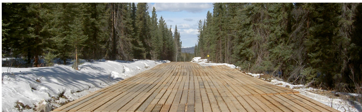
Matted Access Narrowway Road - Southwest of Grande Prairie, Alberta
