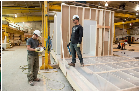
Kamloops Manufacturing Facility, British Columbia
