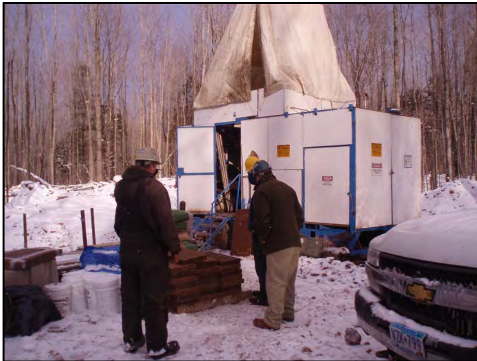
Figure 10.1: Winter drilling at the Section 6 project
