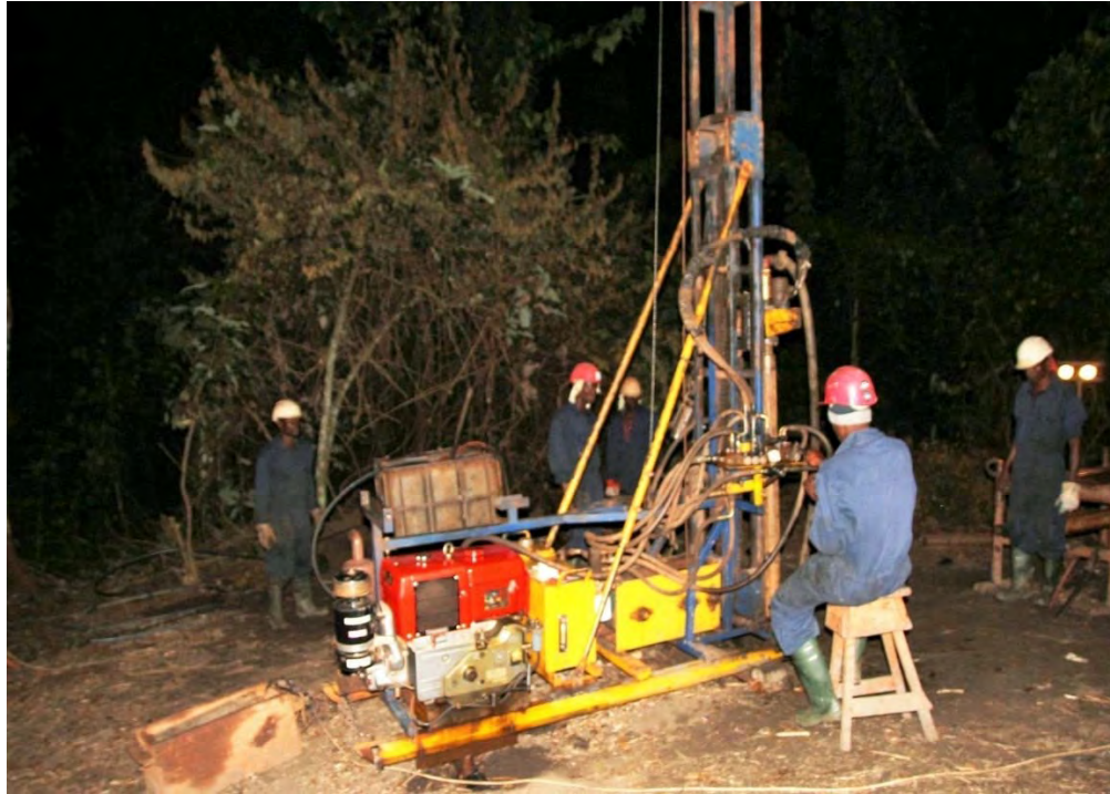
Figure 7: Jacro diamond drilling rig in operation at the Lola Graphite (October 2013).
