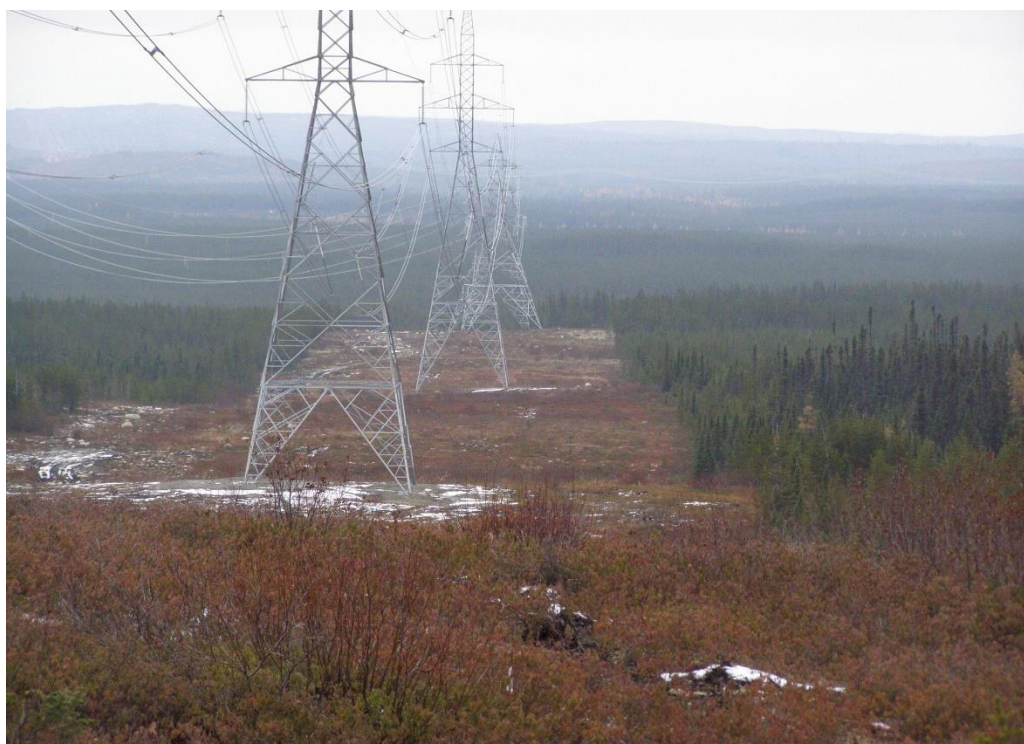
Figure 6 - Power line at Rose Site
