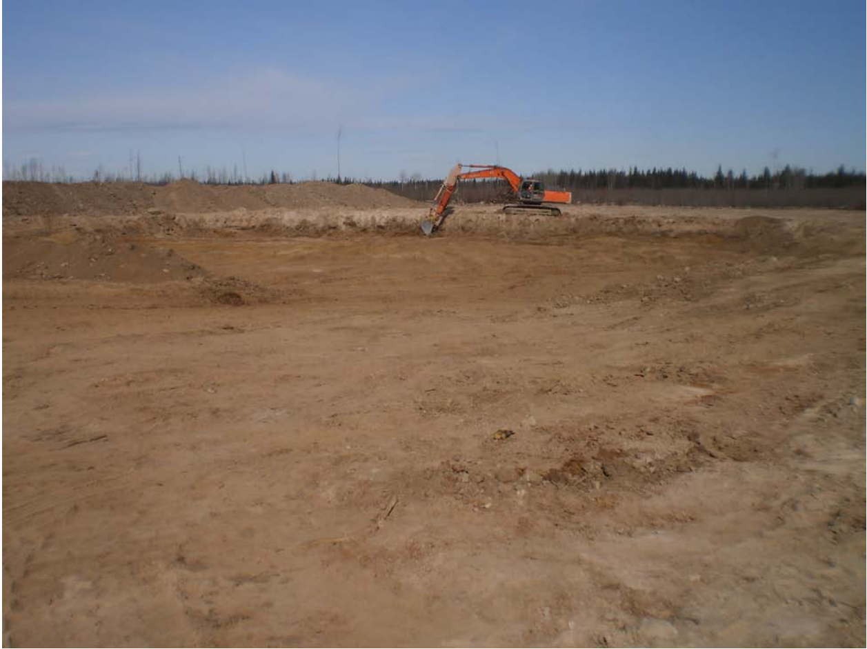
Photo 6 Road material excavation looking northwest from southeast pit edge
