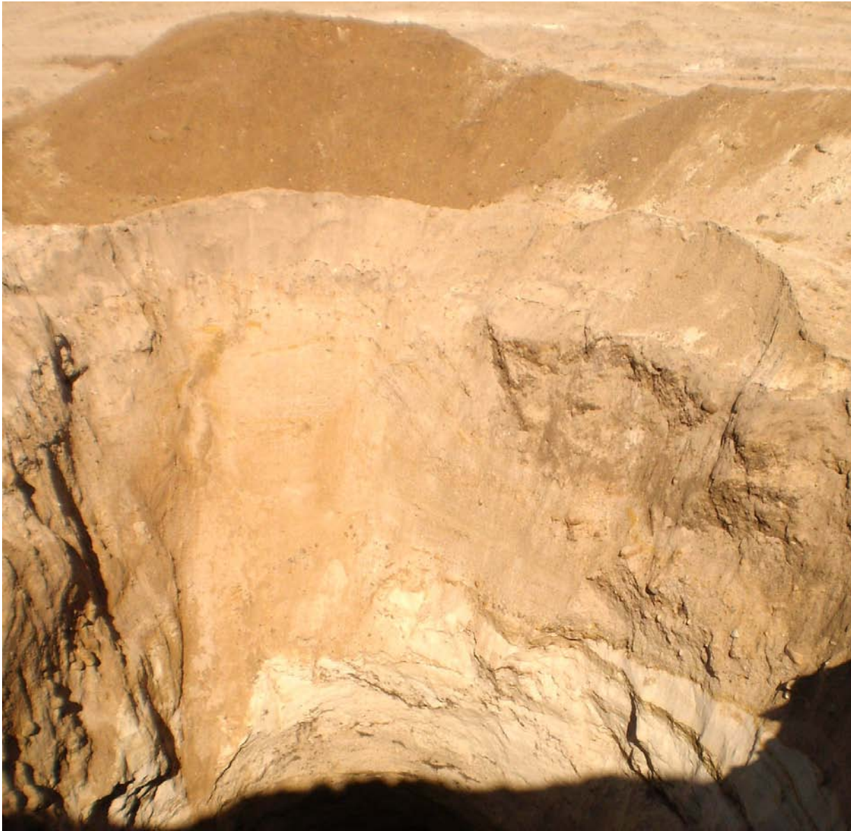
Photo 8 TH321 North test-pit wall (dug on road excavation pit bottom – 3 m below original surface elevation)
