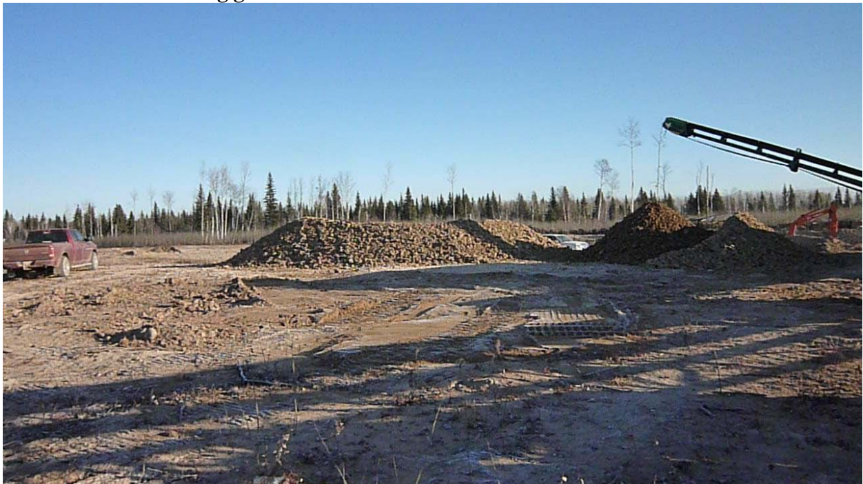
Photo 37 Coarse gravel screened from sand horizon
