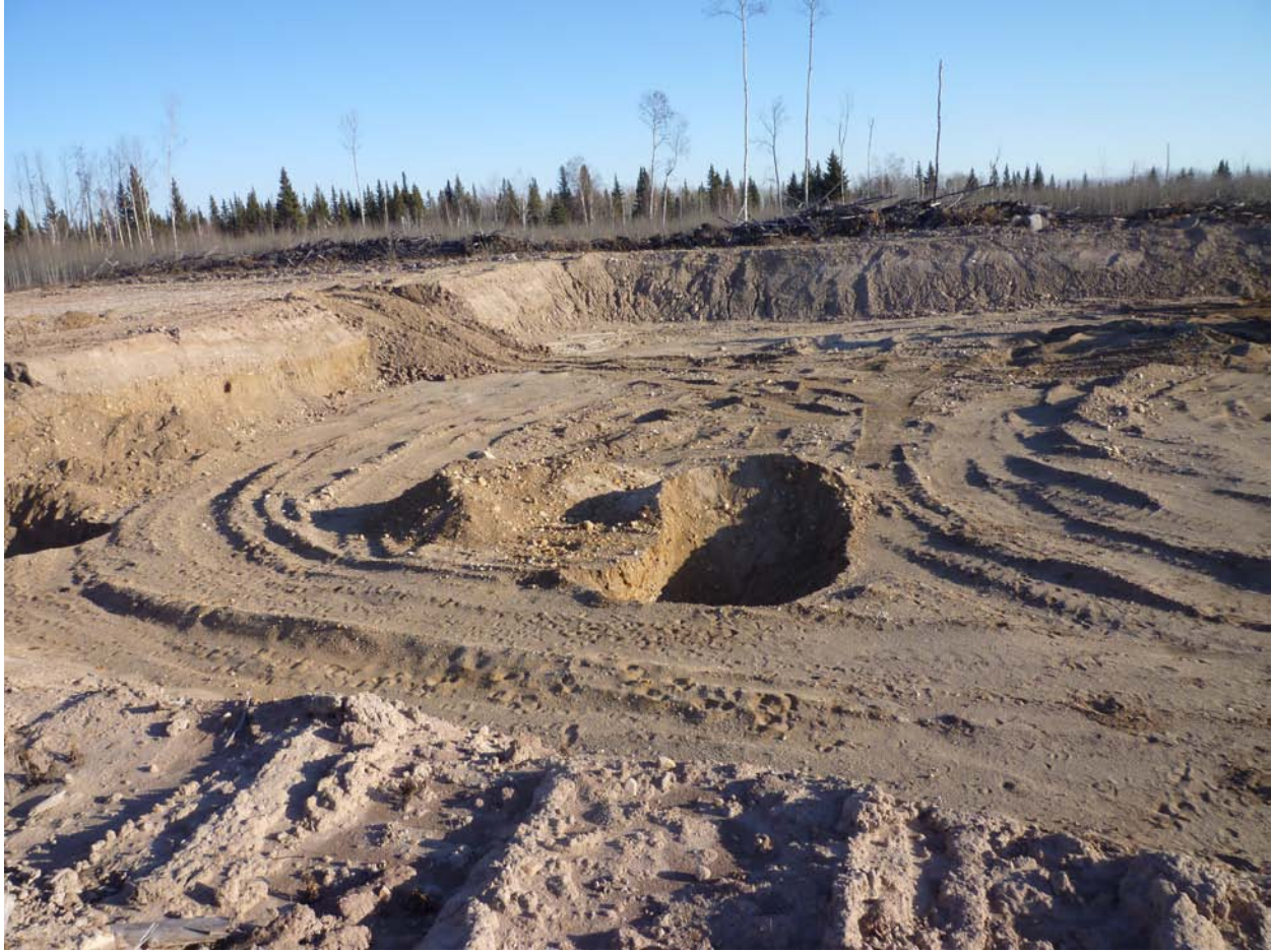
Photo 35 Lease Access Road construction material (mid-lease area)
