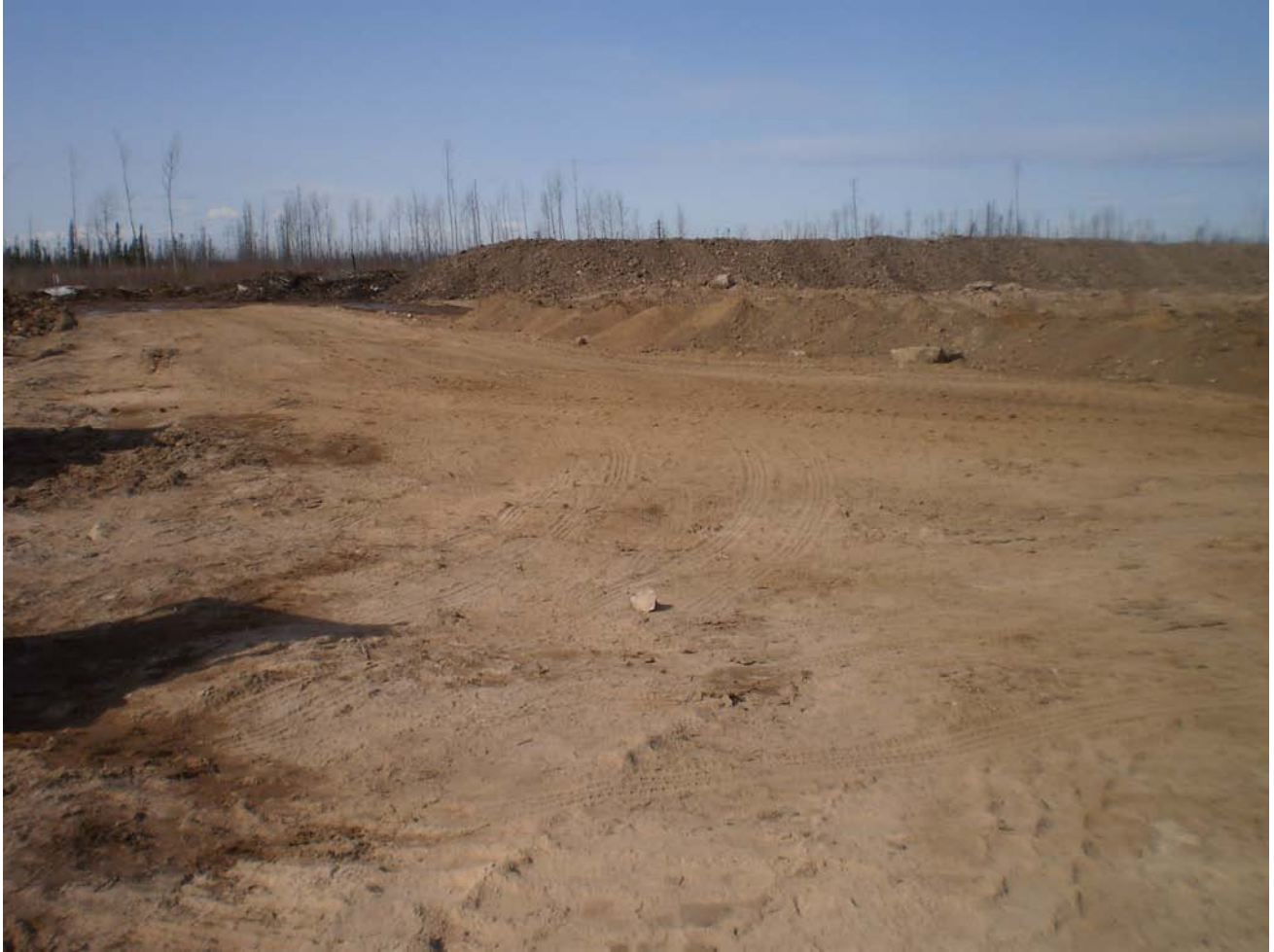
Photo 7 Road material excavation looking west southwest
