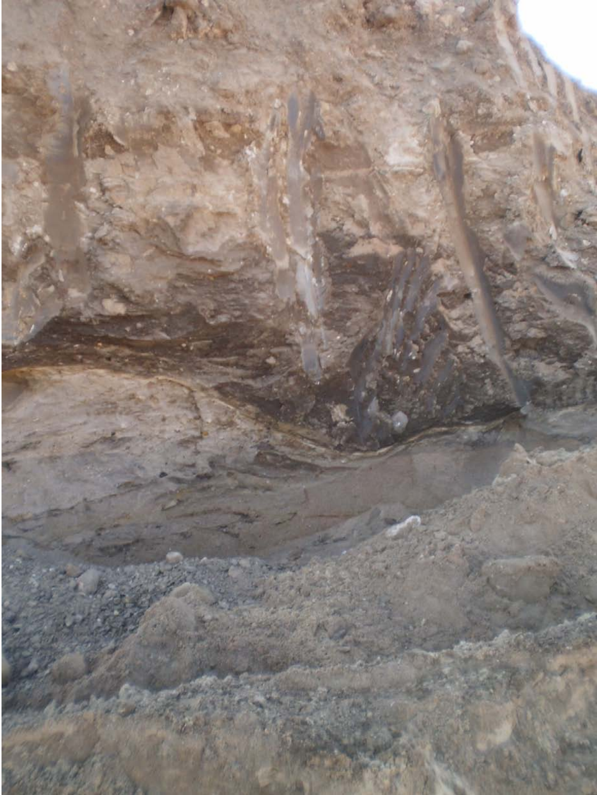
Photo 3` South wall of road material excavation pit
