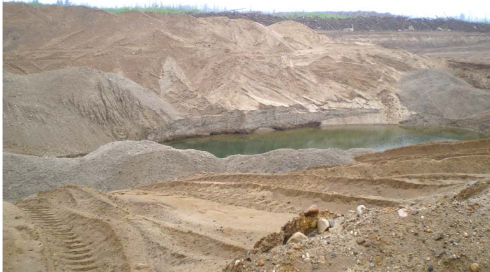
Photo 32 Area where the material for constructing the access road was extracted (mid-lease)
