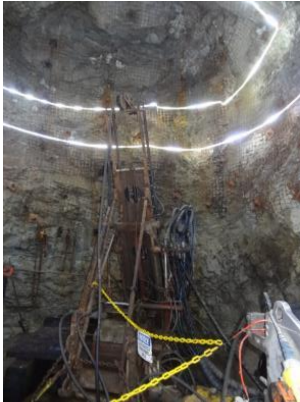
Figure 12.2 Underground Drill Setup on Drill Hole CHQ 1683
