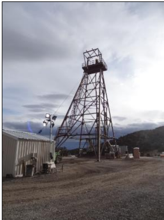
Micon 2022 site visit photograph.
