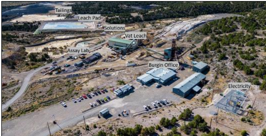
Figure 5.2 Burgin Site Infrastructure
