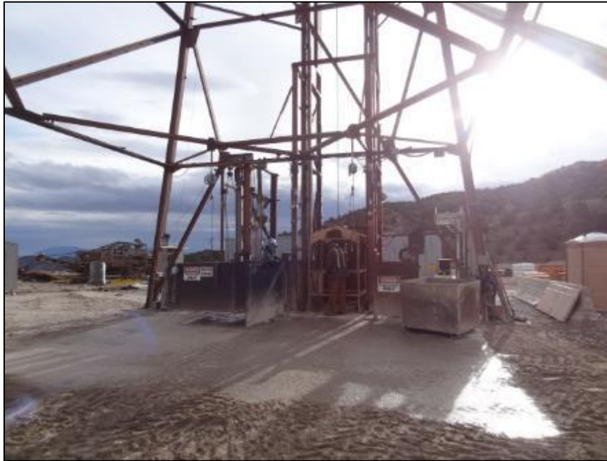
Figure 12.1 Trixie Headframe showing the Cage to Access Underground
