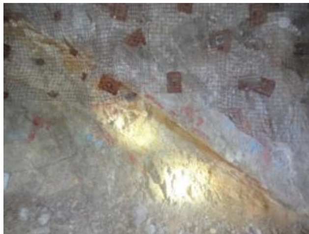
Figure 12.3 Mineralized 45 Fault Zone
