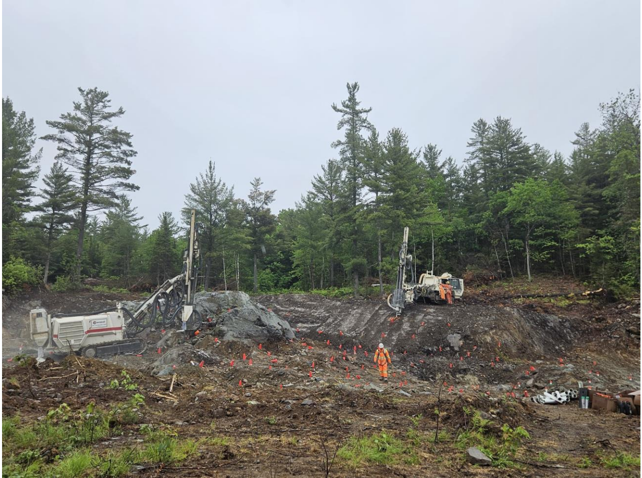
Figure 2. Photo of vertical blast hole drilling of waste on the 007 North Pit.
