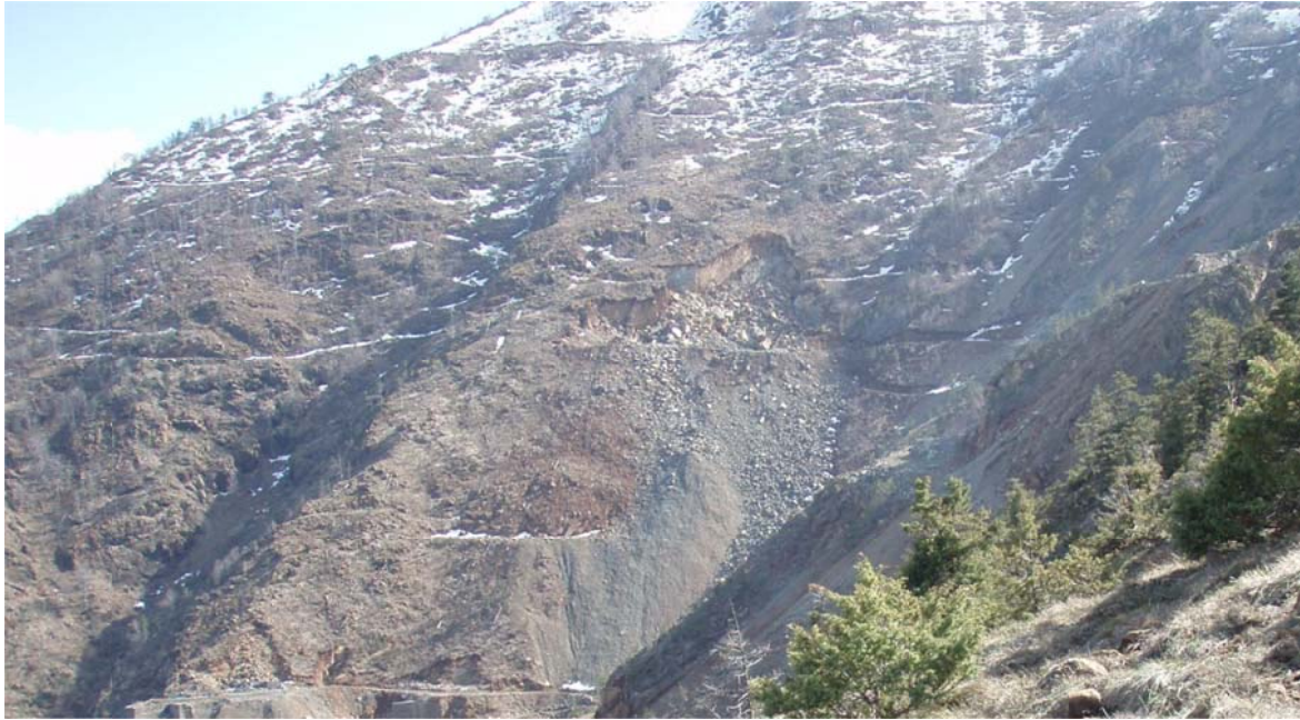
Fig 5 Spoil from Perroi Batres Mine cascading down the slope.
