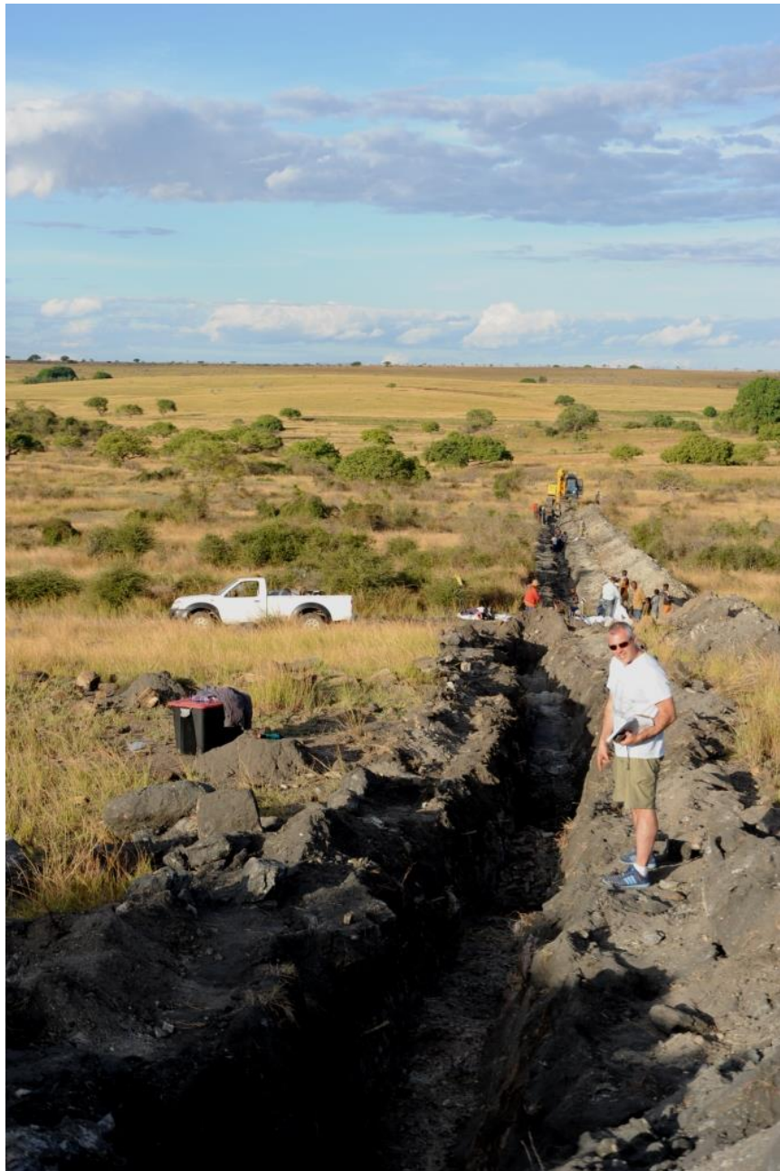
Figure 9-1: Trenching for the bulk sample on Molo, May 2013.
