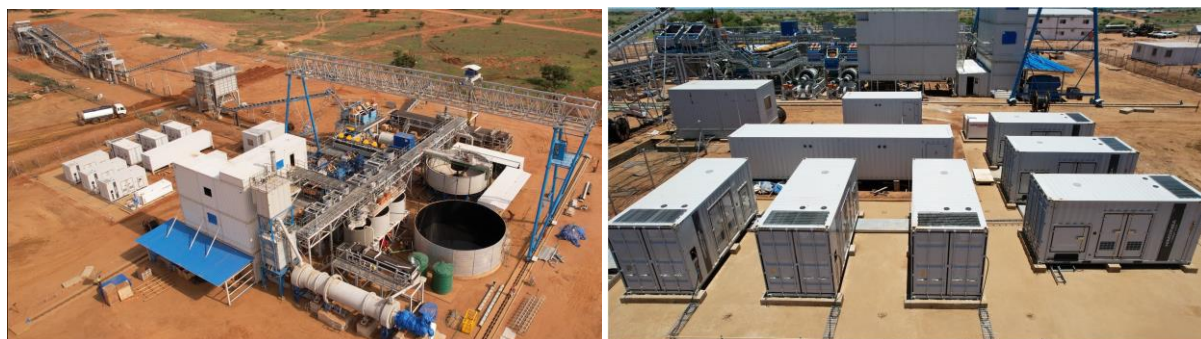
Image: Molo Mine Processing Plant (left) and Thermal Facility (right)
