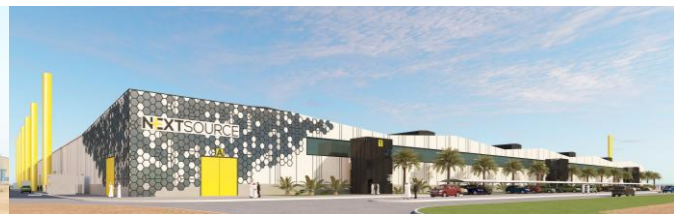
Proposed Renovation of the Building of the UAE BAF
