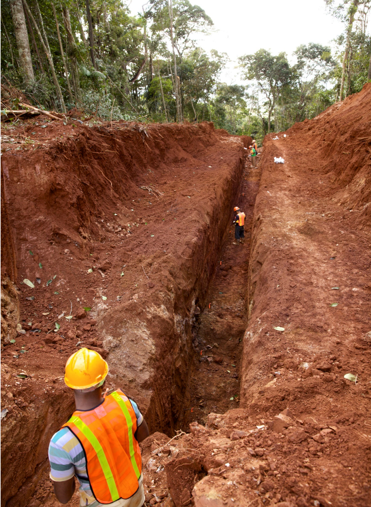
TRENCHING PHOTO TAKEN DURING SAMPLING AND MAPPING
