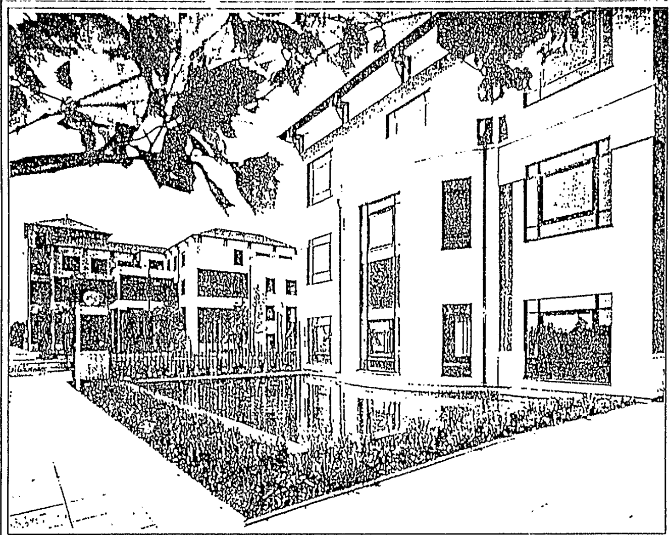
New office development at Wessex Fields, Bournemouth
