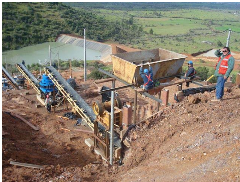
Figure 12-2 General View of Plant Construction
