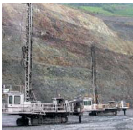
Drill and Blast
