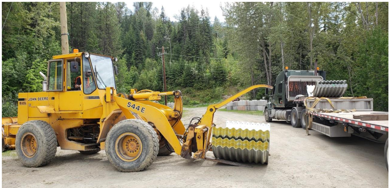
Kenville Mine: steel culvert for new 257 Portal
