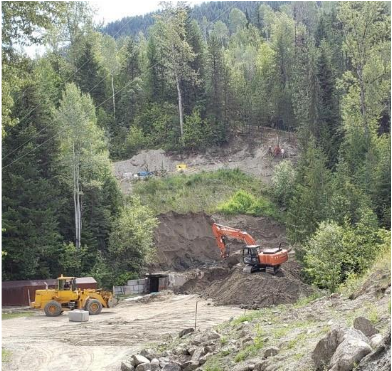
Kenville Mine: 257 Portal initial excavation
