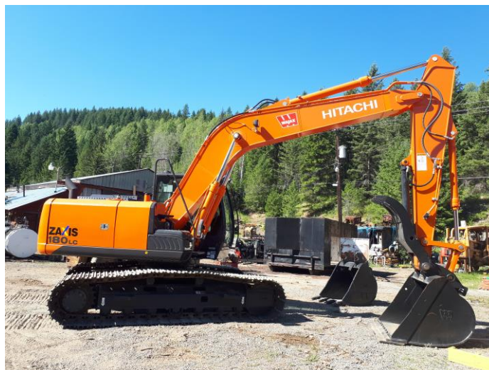
Photo of new Hitachi 180 for Kenville portal excavation
