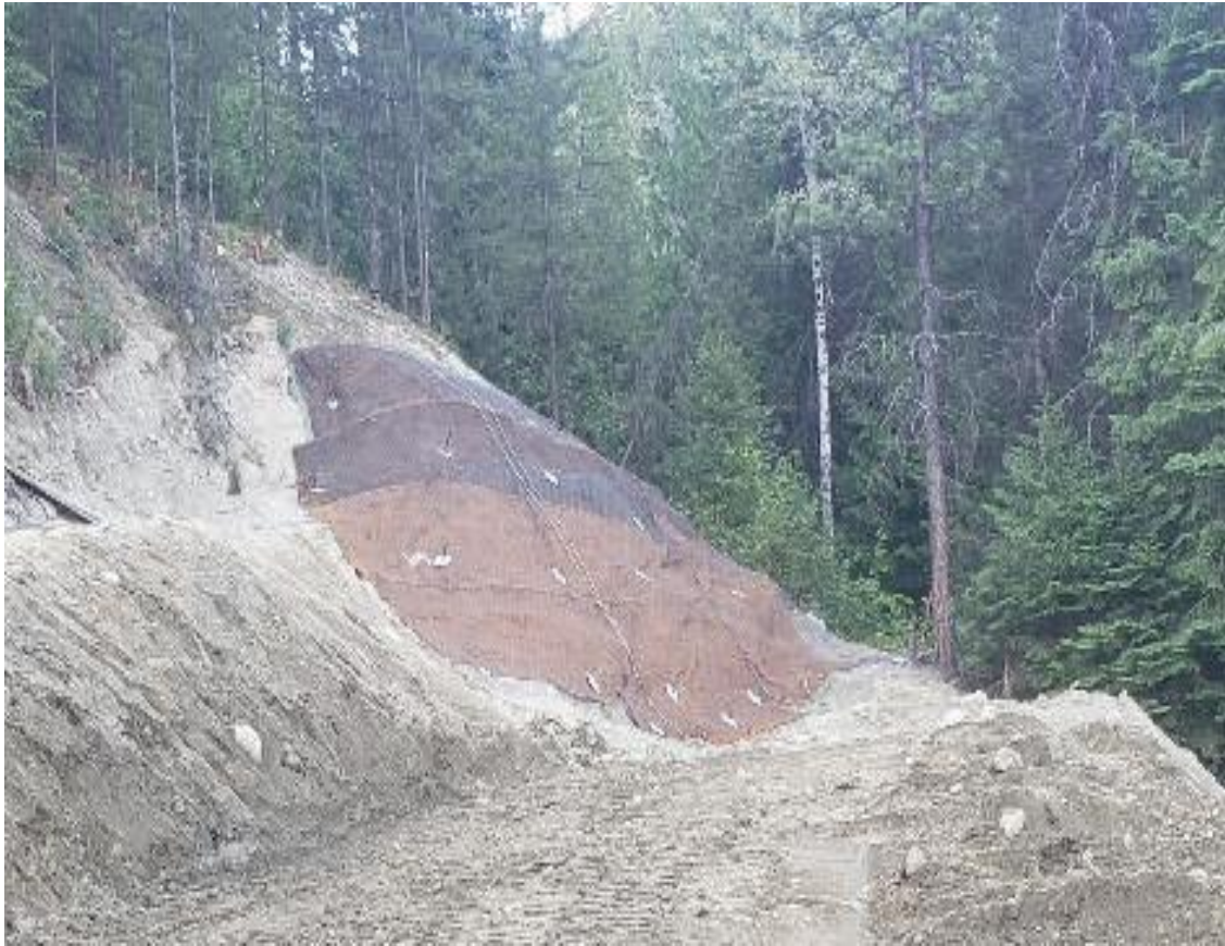
Photo of completely bolted and secured slope above portal site.
