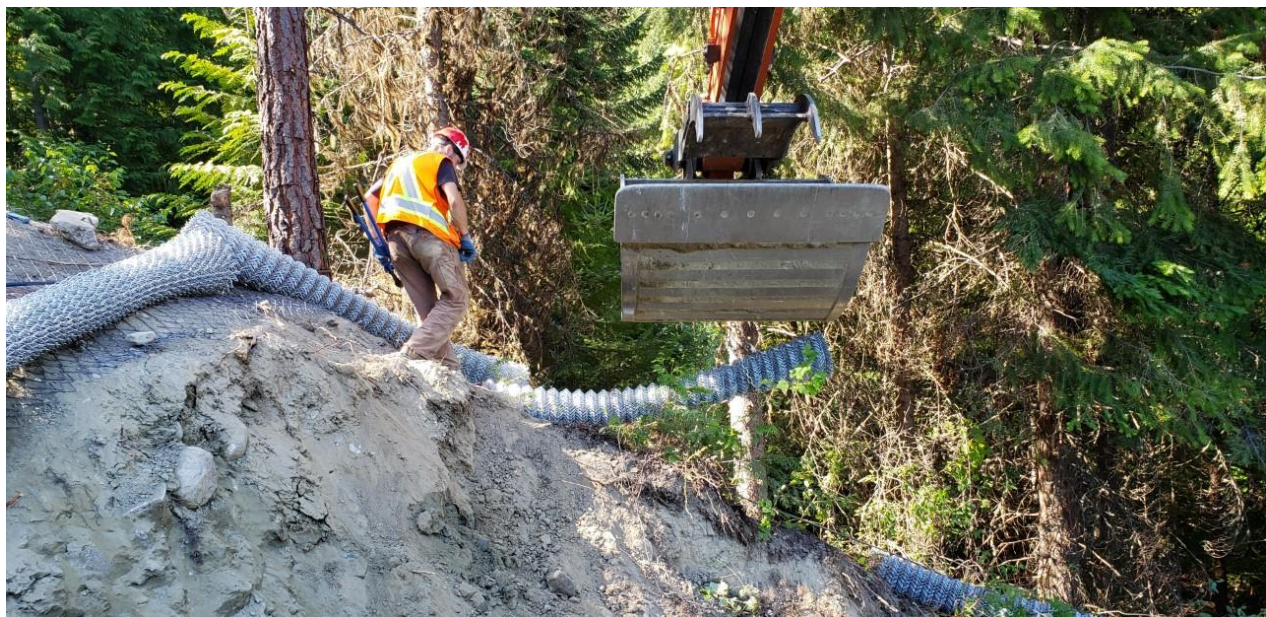
Photo of new screening being placed by Hitachi 180 excavator
