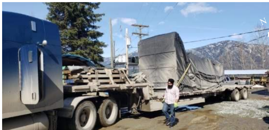
Long anticipated deliver of the Steel Sets for the New Portal Construction
