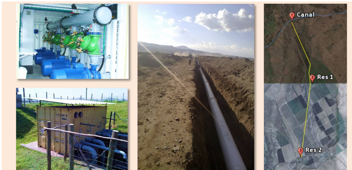
2017 Dejenna chemicals project in Ethiopia - 700 ha of undeveloped land - 4.8 km distance from Irrigation canal to the seconded reservoir -70m difference in ground level
