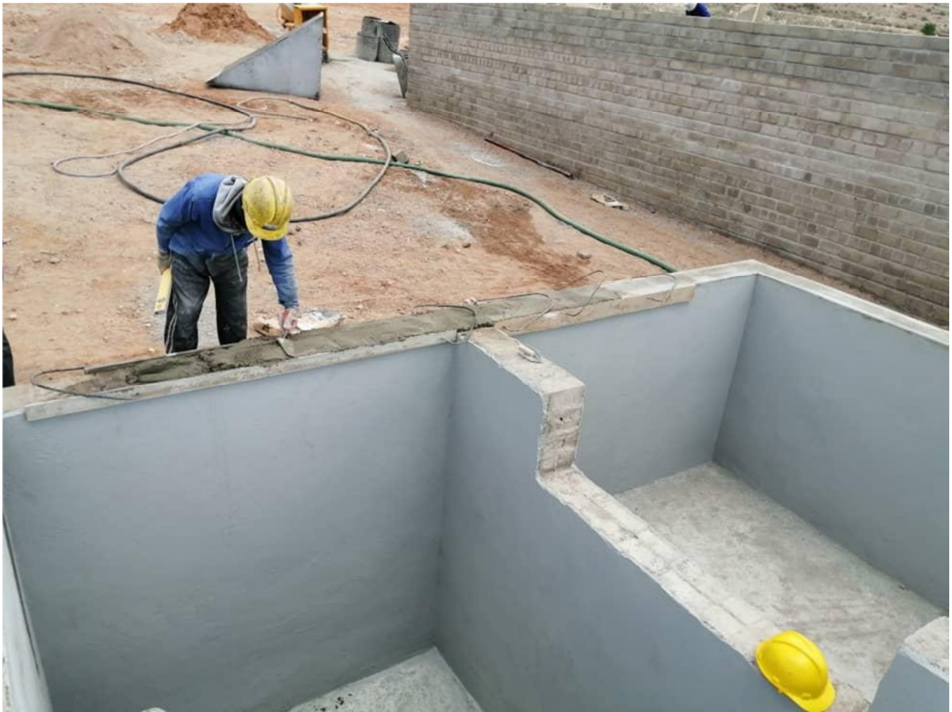
*Above image: Depicts Aukam Team Member sealing the processing plant settling reservoir.
