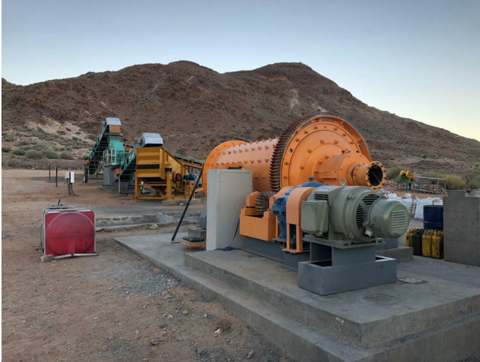
Photo 1 showing commercial scale rod mill, screeners and conveyance systems
