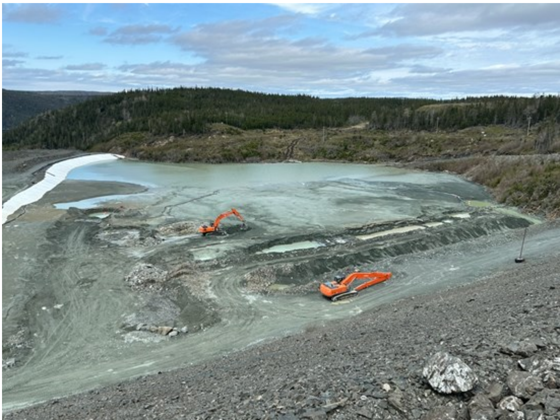
Figure 3. TSF2 Tailings Facility
