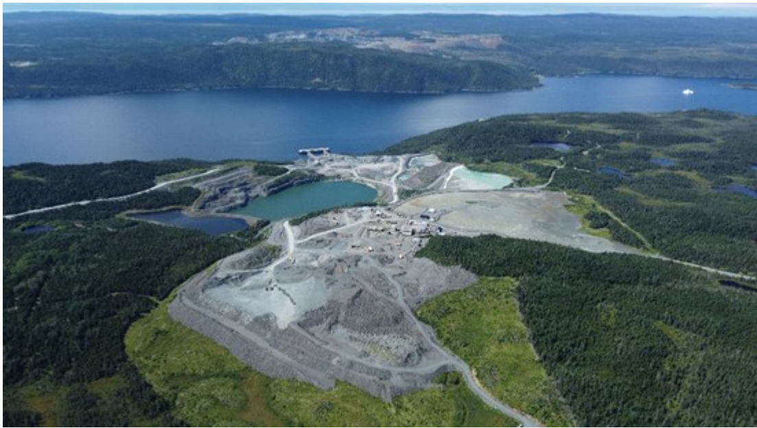
Figure 3. Pine Cove Mill Facility
