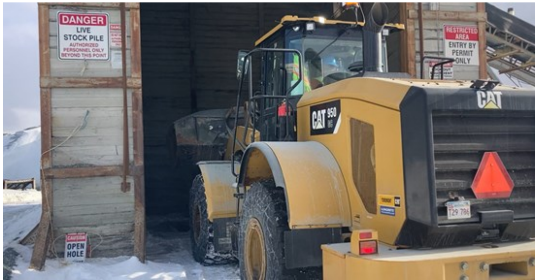
Figure 3. Loading Crushed Mill Feed
