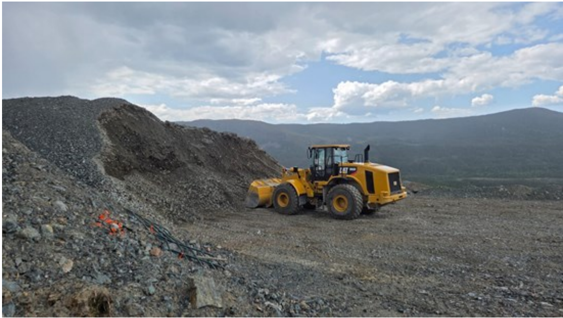
Figure 1. Excavating the historic Richmond Mines ore pad
