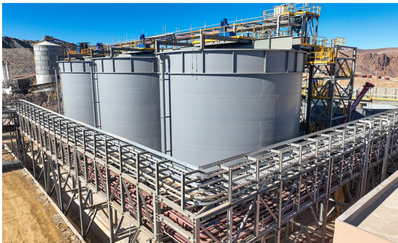
Figure 1 – Completion of Leaching Tanks at Zgounder
