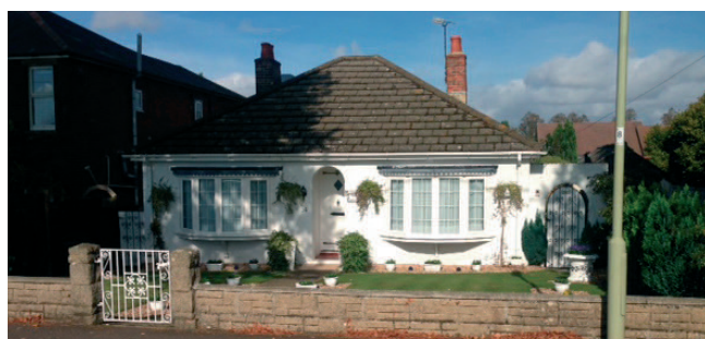
54 Grange Road, New Arlesford
