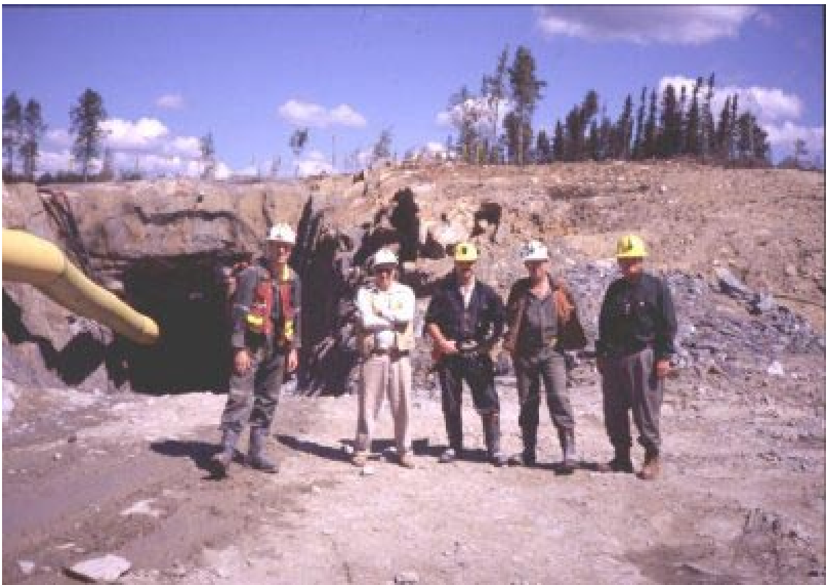
Figure 6-1. Portal/decline access to the Thunder Lake Deposit Main Zone gold mineralisation for bulk sampling; 1998 Teck Cominco and Corona Gold joint venture (MNDM, 1998).
