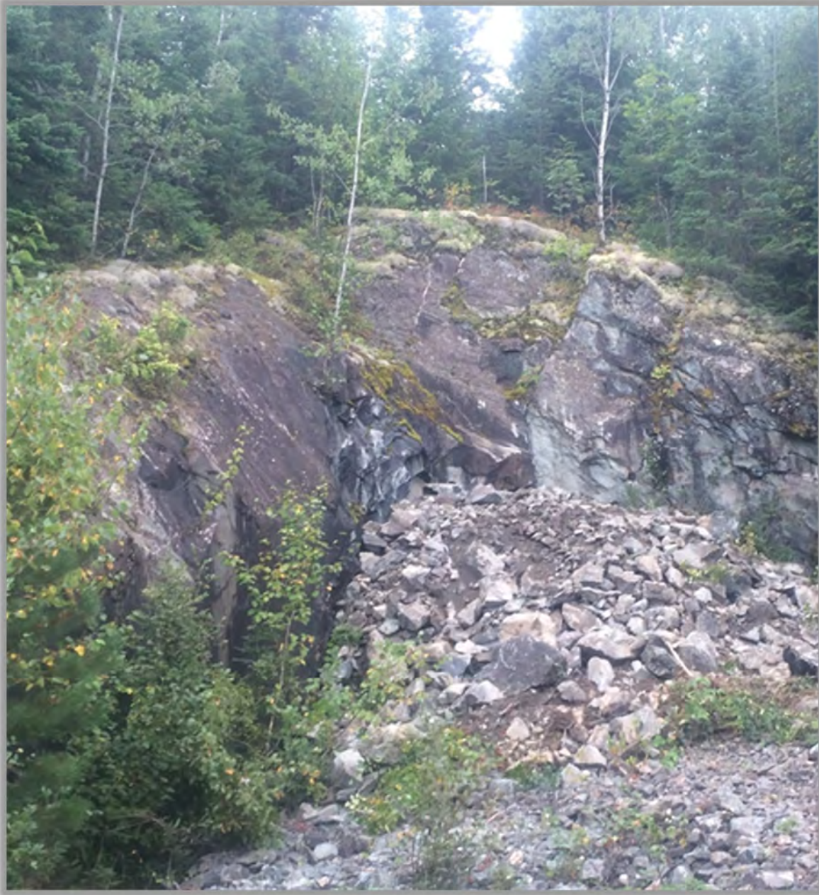
Figure 5.4 Current Condition of the Sealed Portal
