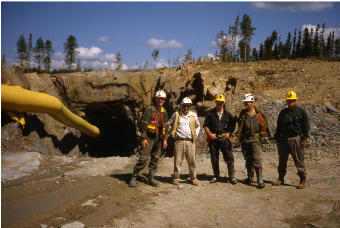
FIGURE 6.1 PORTAL/DECLINE DEVELOPMENT ACCESS TO MAIN ZONE GOLD MINERALIZATION OF THE THUNDER LAKE GOLD DEPOSIT
