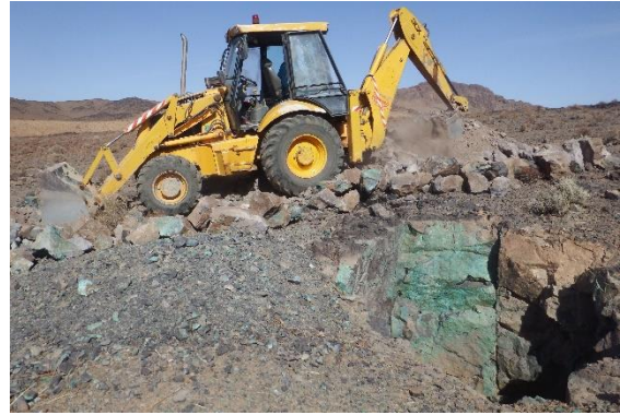
Trenching at Agdz
