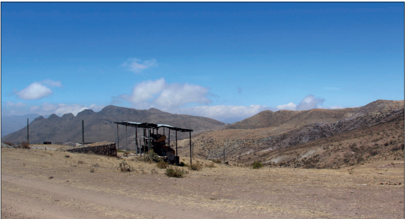
Figure 3: General view of the 30 tonne / day crushing plant. The plant is permitted but has not been used for several years.
