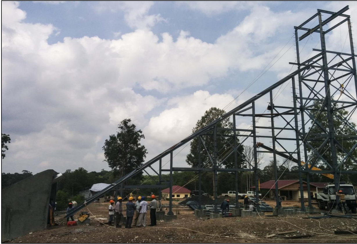
Figure 2. Phum Syarung Site showing incline with head frame, laboratory and field office.
