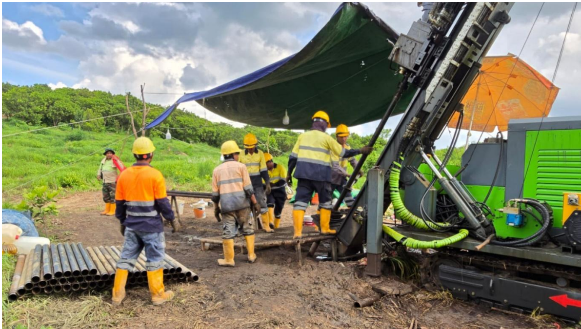
Figure 1 Mobilizing Drilling Rig for Andong Bor
