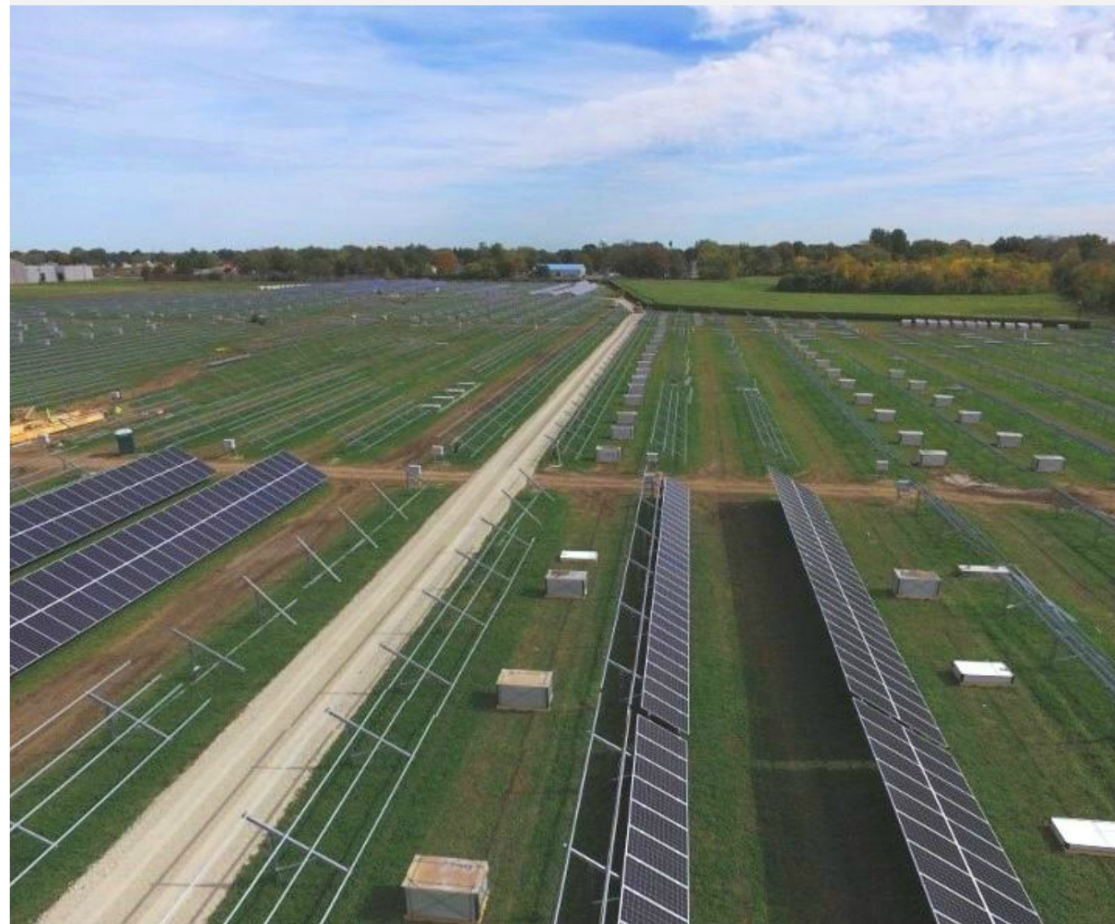
ALTERRA'S KOKOMO SOLAR PROJECT UNDER CONSTRUCTION
