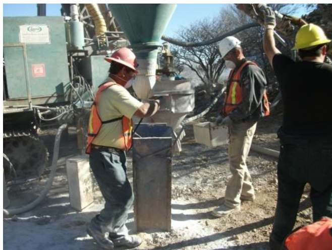
Figure 25. Sample splitting.
