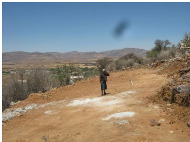
Figure 30. Clean Drill Pad.
