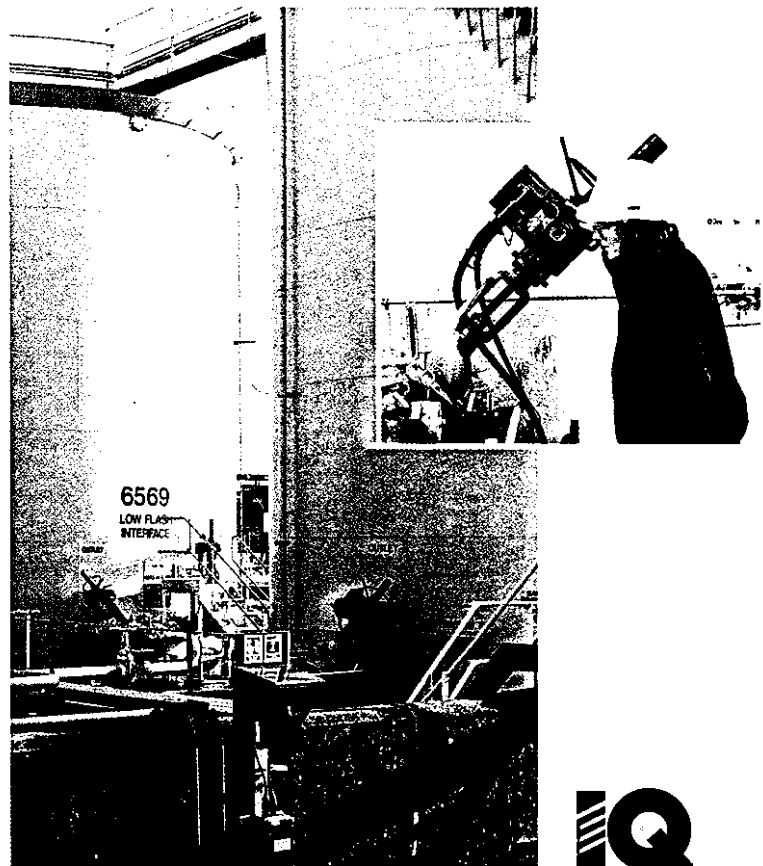
Above: the hand held IQ Communicator provides event monitoring and diagnostic facilities for the IQ range of electric valve actuators.
