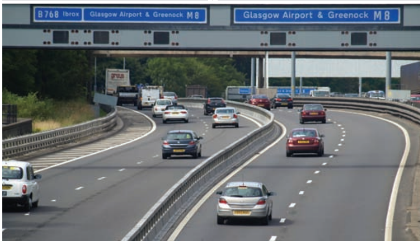
New separation barrier for the M8 Glasgow.
