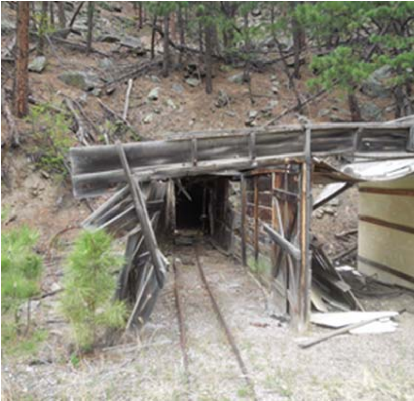
Figure 16: Bullion Mine Adit (as at May 2012)
