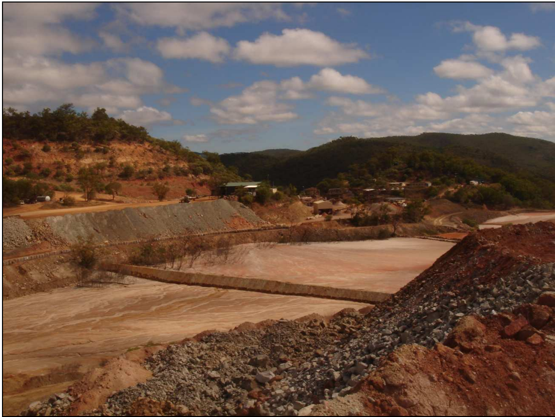
Figure 17-3. Tailings Disposal Area
