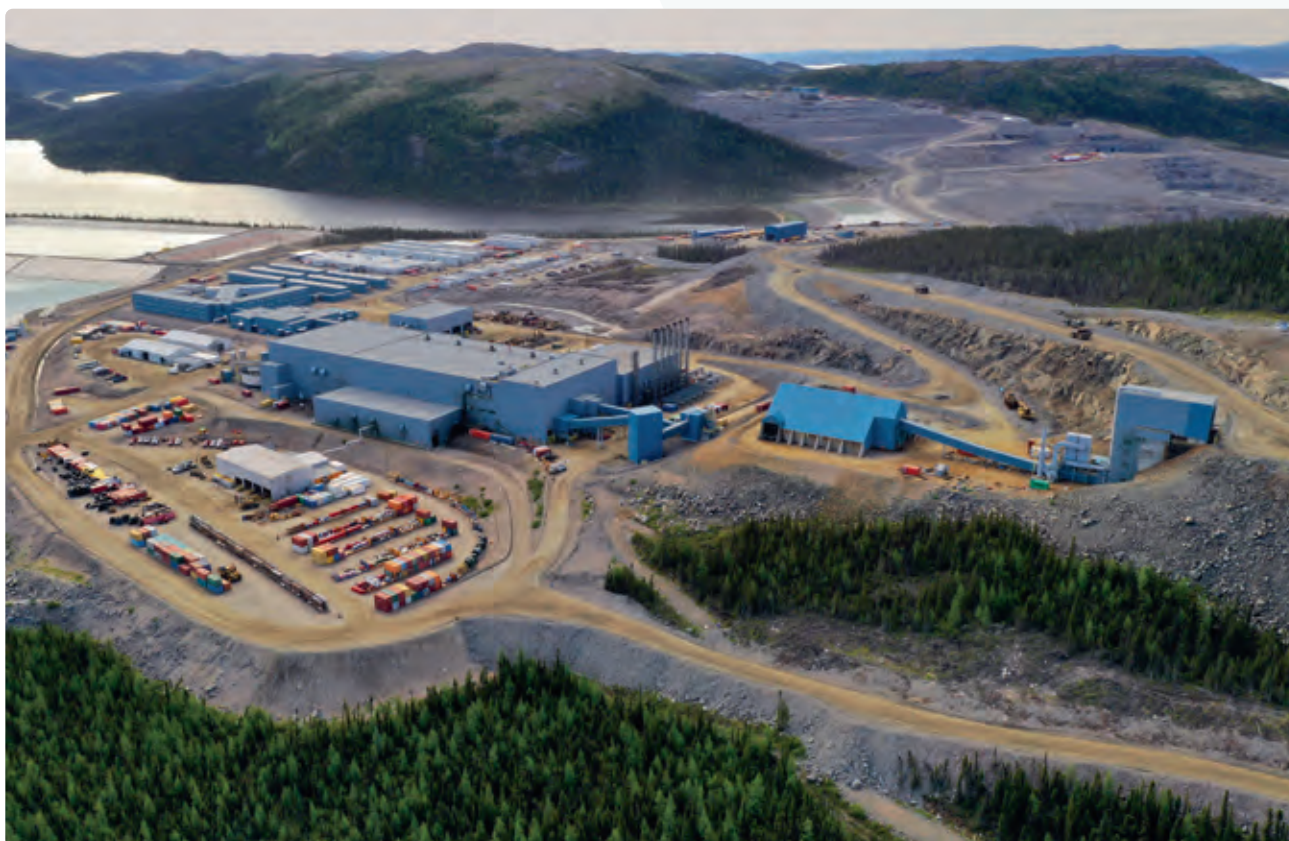
Vale - Voisey's Bay mine
