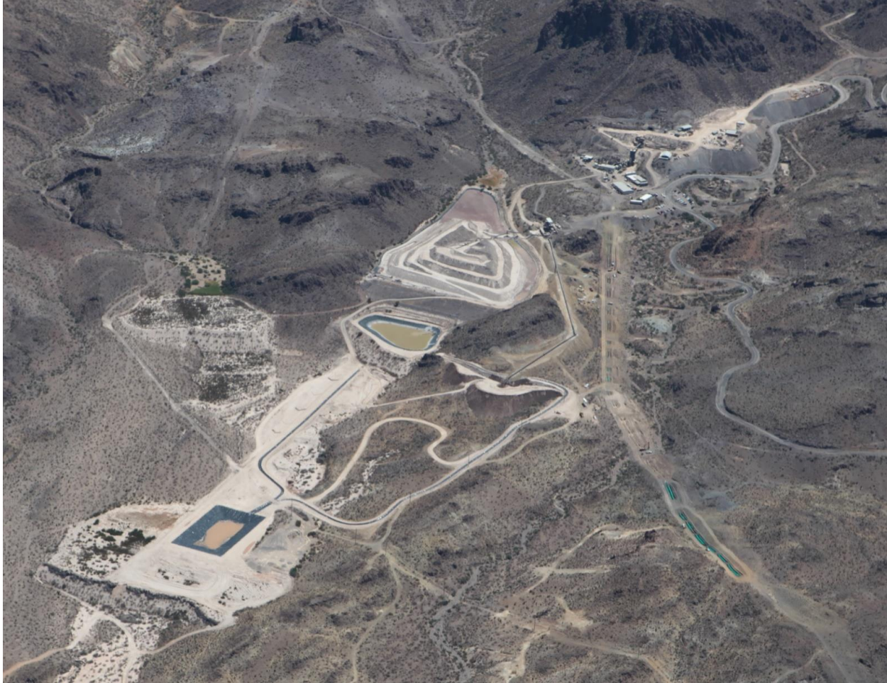
Gold Road Property showing the Mine Entrance, Mill and dry stack tailings
